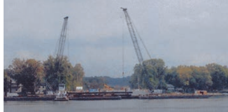
Walsh/Vinci-JV on the East End Bridge Crossing
