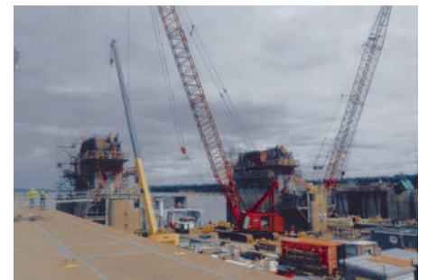
4100 Crane Operators Brad Davis and Steve Shepard at Olmsted Dam
