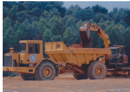
New Apprentice Russell Story trying out the Excavator while loading the Articulating truck during orientation
