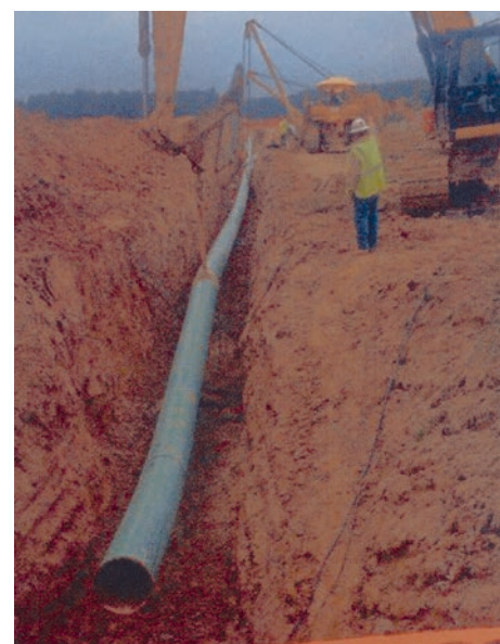
Precision Pipeline on the Indiana & Ohio Atec pipeline job
